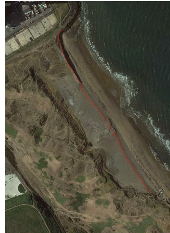
Figure 5 – Baseline cliff top survey (South)
